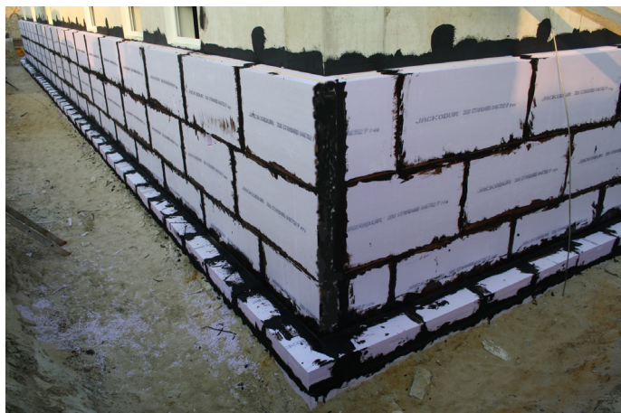
Photo: Installing perimeter insulation in pressing water (groundwater)
