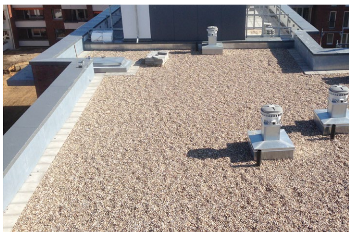
Inverted roof, gravel-covered
