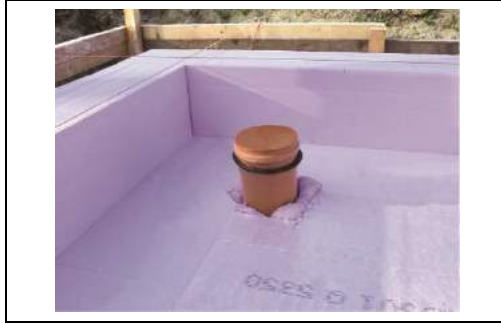
Figure 9 Installation of penetrations
