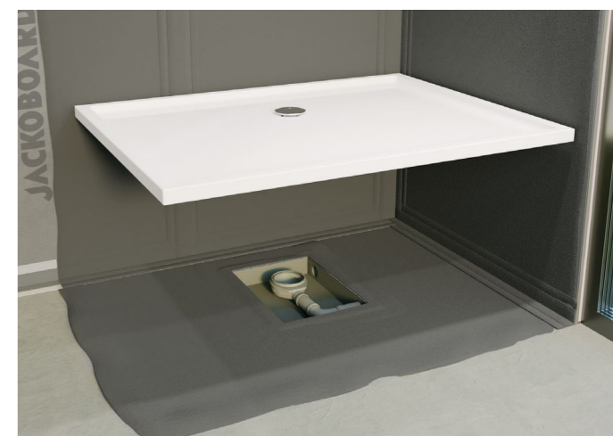
4) Insert the drain and shower element
