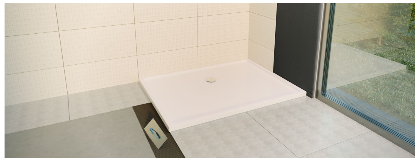
5) Tile the walls and floor
