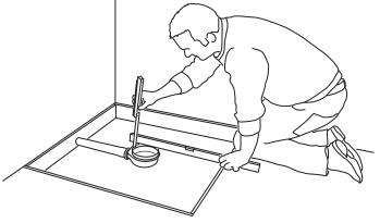
2) Position the drain at exactly the right height. The height difference between the upper edge of the drain and the level of the screed depends on the thickness of the shower base (see distance A – C in drawing and table on page 6).
