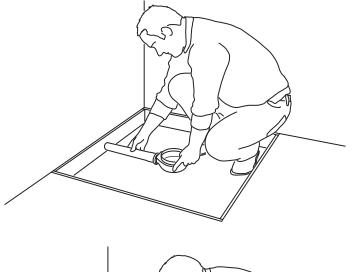
1) Push the drain outlet into the existing DN 50 pipe and centre it. The supplied drain has a DN 50 pipe connection. For connection to pipes in 2" or 1½" is a suitable adapter necessary.
