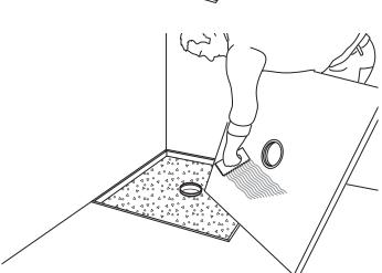
**4)** Once the levelling screed has cured, apply cement-based flexible tile adhesive with a notched spreader to the entire underside of the shower base.
