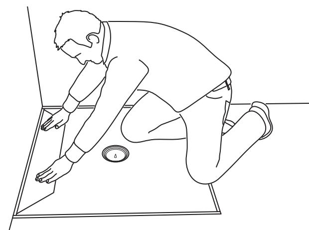
**8)** Position the pipe duct element (2) in the screed recess and press firmly into place. BOARD-FIX® (6) special adhesive and sealing agent guarantees the durable seal integrity of the bond.
