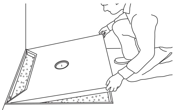
**4)** Connect the drain nozzle on the shower element (DN40) to the on-site drainpipe.
