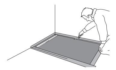
**8)** All connecting joints are sealed with the JACKOBOARD<sup>®</sup> sealing set 2-k (or equivalent).
