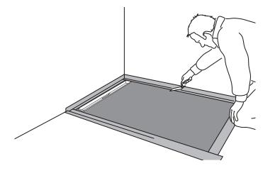
**9)** All connecting joints are sealed with the JACKOBOARD® Sealing set 2-k (or equivalent).
